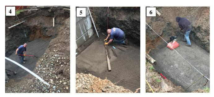
The hole is then extended westward to allow for the installation of the third septic tank. Photo 4, 5 and 6 show the raking, leveling and compacting of the tank floor to the elevation necessary to continue fluid flow from the second tank influent (+79" to invert).
