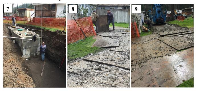
Final elevation checks before placement of the third tank are performed, as shown in Photo 7. Then placement and shifting of 1" plywood boards must be done to provide adequate traction for truck and boom, as seen in Photos 8 and 9.
