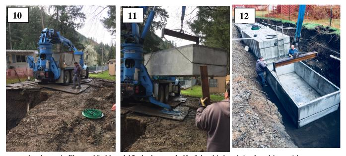
As shown in Photos 10, 11 and 12, the bottom half of the third tank is placed in position and aligned according to field measuring and painted markers.
