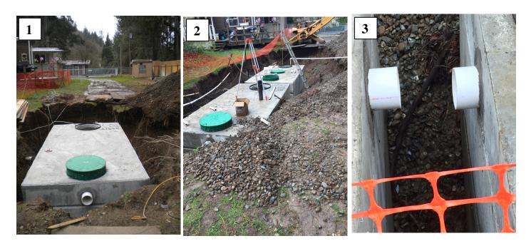
Photo 1 shows the single 3000 (approx. 3095 capacity) concrete septic tank, placed and leveled. Photo 2 shows the Site after the second tank is placed. Photo 3 shows the alignment (effluent of eastward effluent into influent of west-adjacent septic tank). These two will accumulate most solids over time.
