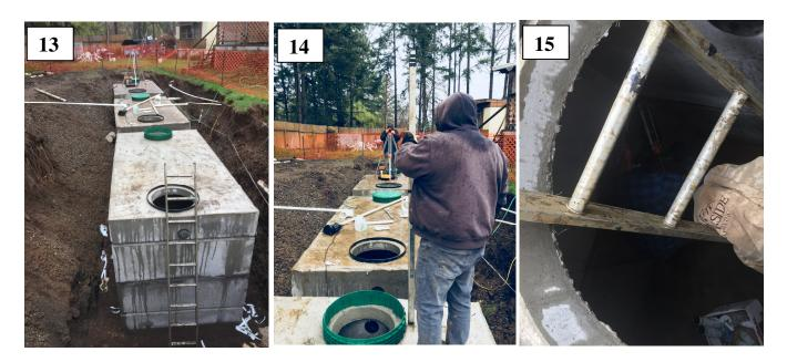
Similarly, the top half of the septic tank is placed, correct elevation of the third tank assured, and interior sealing between top and bottom tank halves is completed (Photo 15). After each of these tank installations, before excavation for the next tank, each tank is filled with water to above the tank seam to assure tank tightness.
